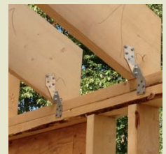
Hurricane clips on roof trusses
