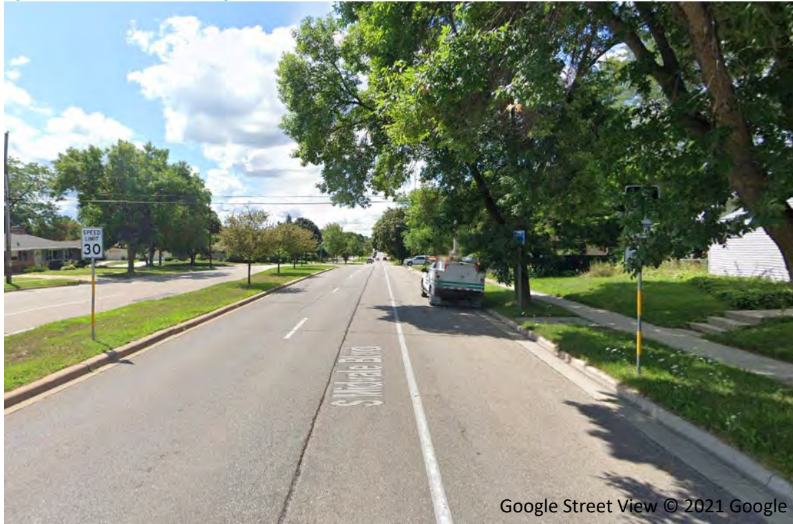
Figure 4 South Midvale Blvd (Wright St/Fair Oaks Ave to STH 30) – three travel lanes, bike/parking lane, median
