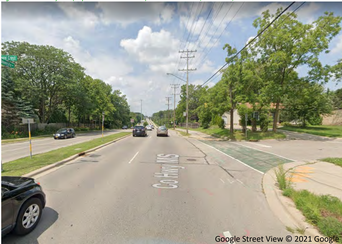
Figure 10 University Ave (Capitol Ave to Allen Blvd) – two travel lanes, bike lanes, median
