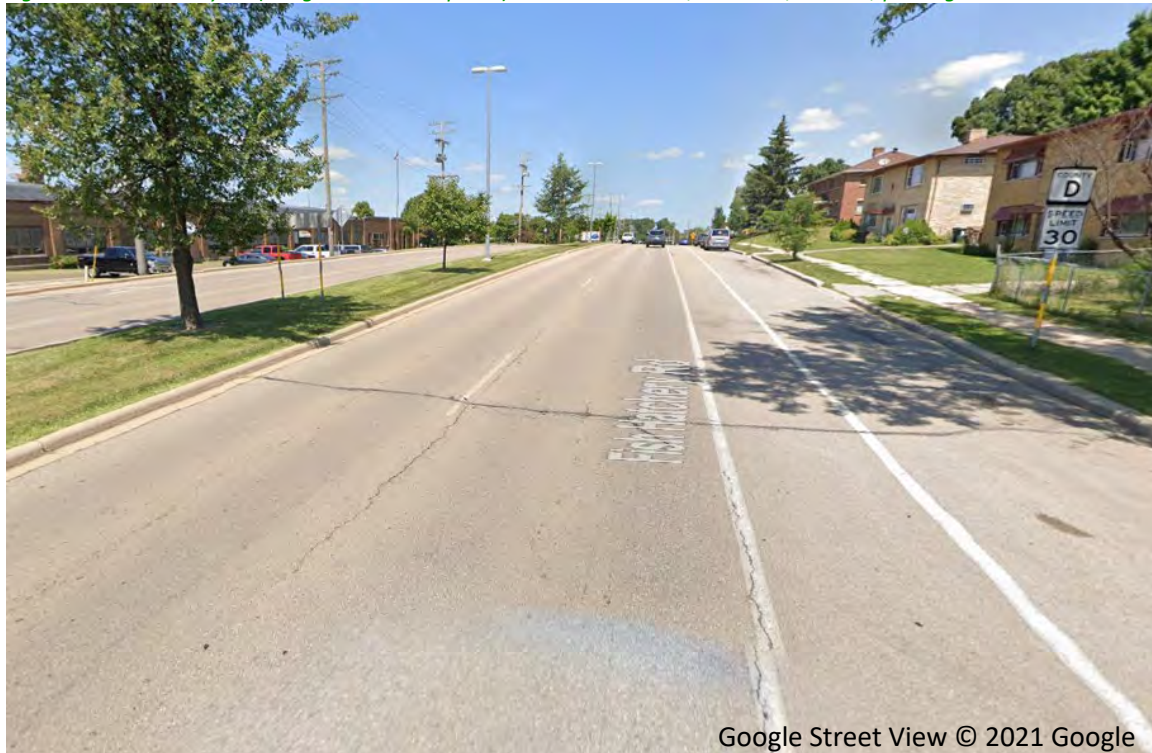
Figure 5 Fish Hatchery Rd (Badger Rd to Catalpa Rd) – two travel lanes, bike lane, median, parking lane
