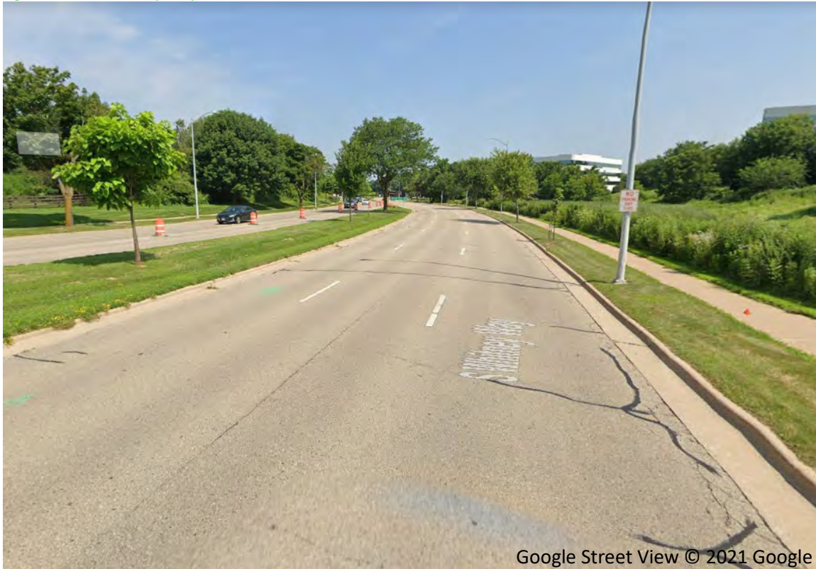
Figure 9 South Whitney Way (Science Dr to Mineral Point Rd) – three travel lanes, median
