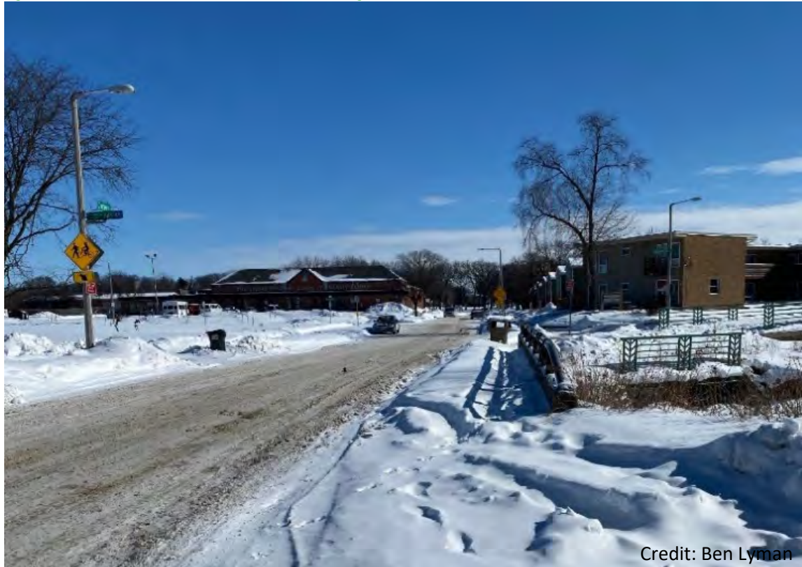
Figure 17 Snow Covered Sidewalk - Darbo Drive Bridge at Starkweather Creek, Madison
