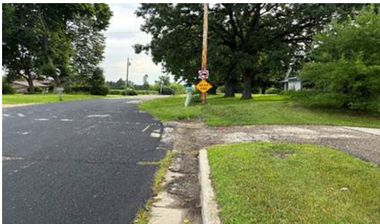
1: Urbanized section at Johnson Health Tech looking east
