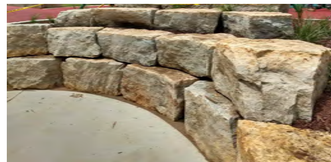
STACKED STONE RETAINING WALL
