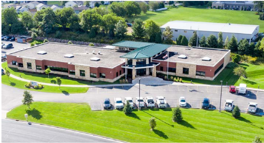
Landmark Services Cooperative headquarters; photo by Robert Bertera
